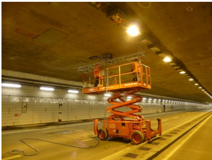
Figure 4: Examination of a tunnel ceiling.
