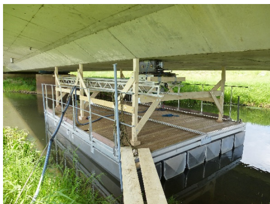
Figure 6: Examination of a prestressed concrete bridge with the help of a floating platform.
