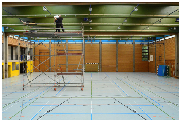
Figure 7: Examination of prestressed concrete girders in a sports hall.
