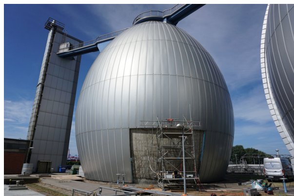
Figure 7: Examination of tendons of a digester.
